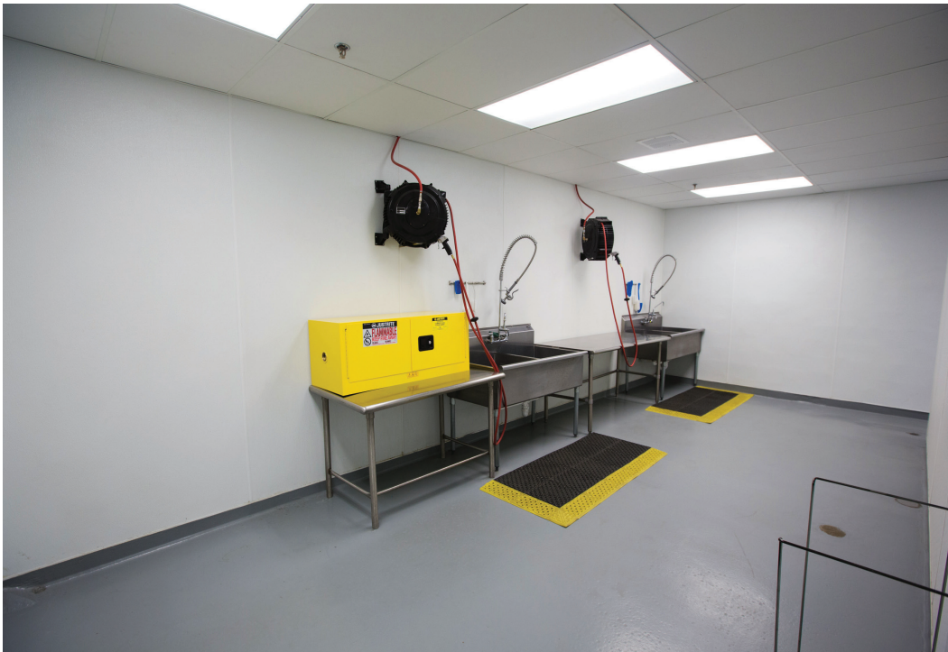
GROUND FLOOR CLEAN ROOM
